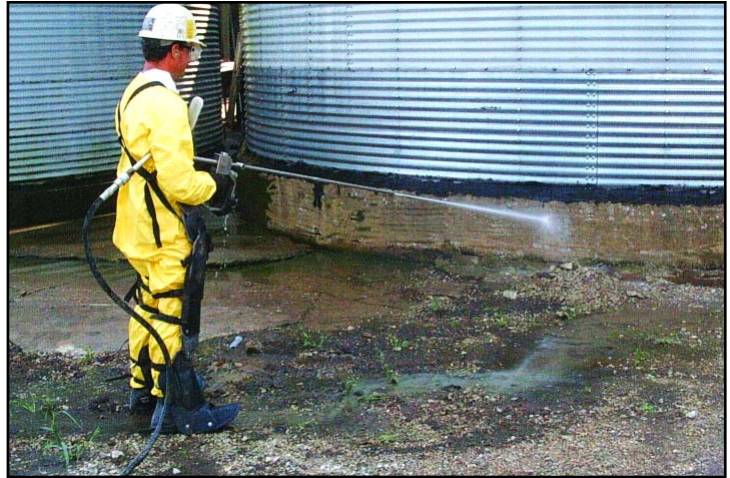
Water blasting is being used for a wide variety of services.
